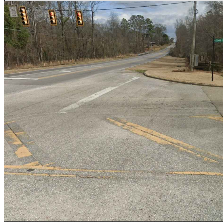
2. At Lodge Drive and Vaughn Road Facing East
