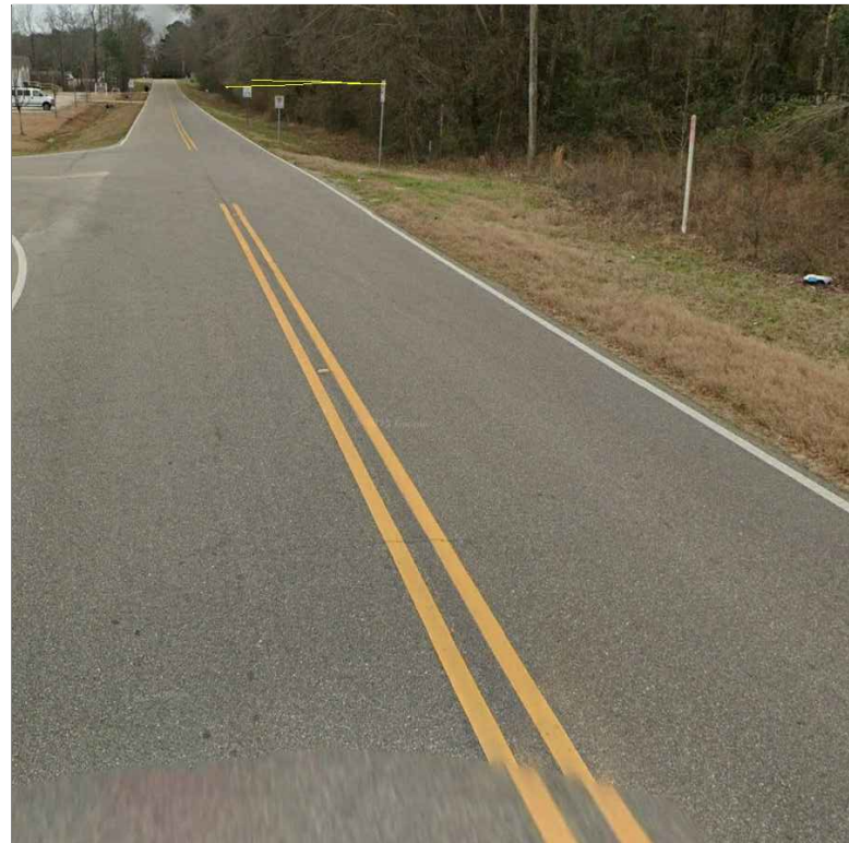
10. Antioch Lane at Georgia Washington Road Facing East
