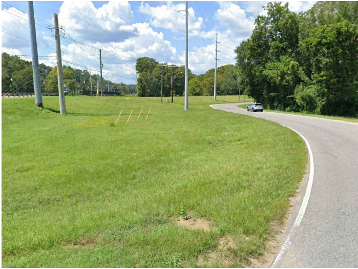
No. 2 - Looking West along Lower Kingston Road
