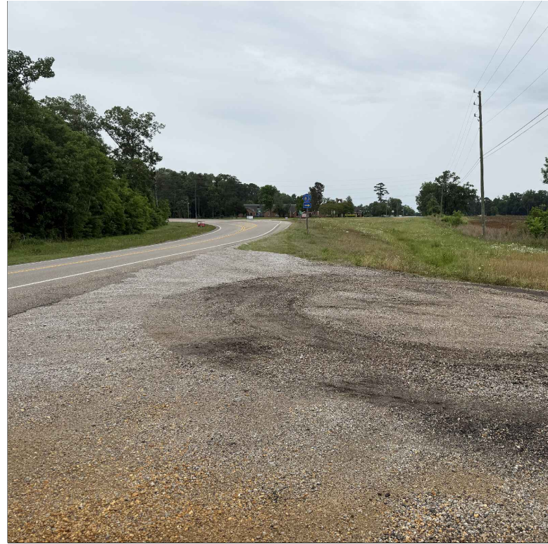
7. Vaughn Road at Proposed Trail Route Facing South toward Wallahatchie Road
